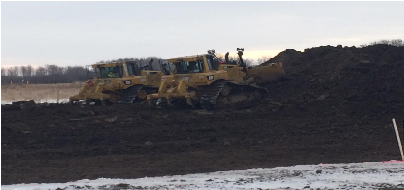
806 + 140 East side of the Pipestone Creek Dozers tandem pushing topsoil
