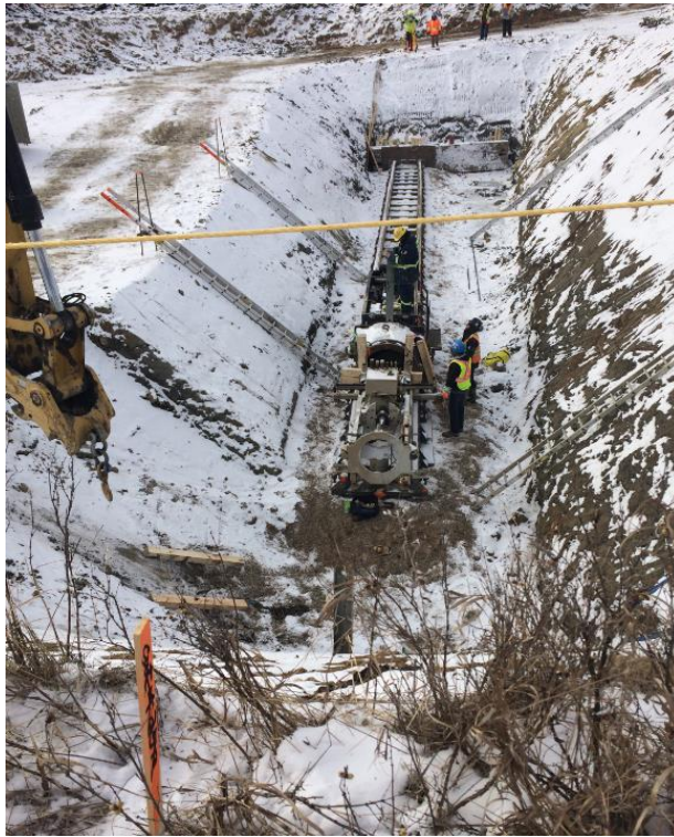
805 + 420 Track bore East side of the Pipestone Creek
